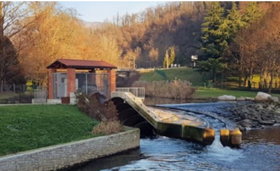
Besozzo (VA) "Folla" Plant - 65 kW
