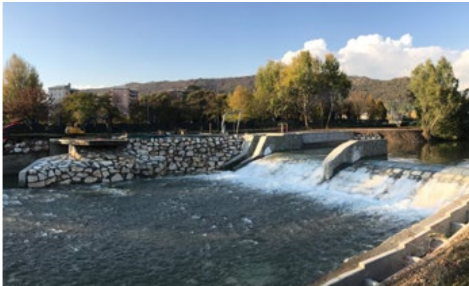
Brescia - "Urago" Plant - 400 kW
