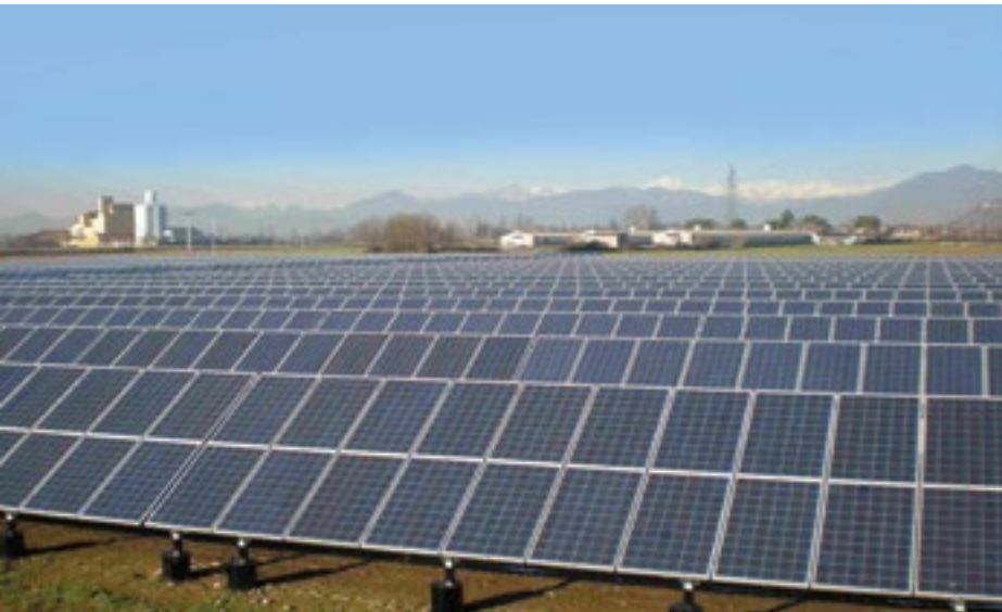
Impianto FV "Cologne" (BS) - 990 kW
